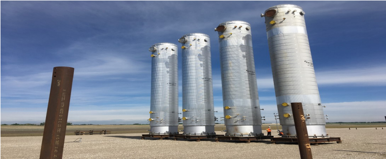
Canada - Custom steel grillage eliminated concrete.
