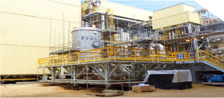
Russia - Process module supported on helical piles.
