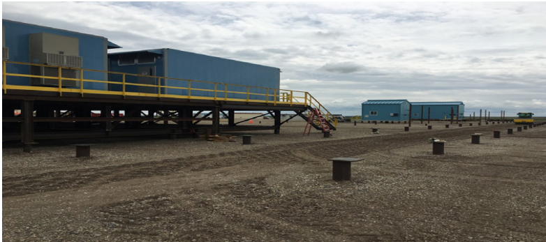
Canada - Elevated, modular buildings supported on helical piles.
