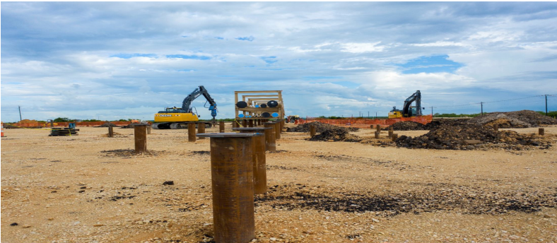
Texas - Helical piles expedited construction of this modular piperack.
